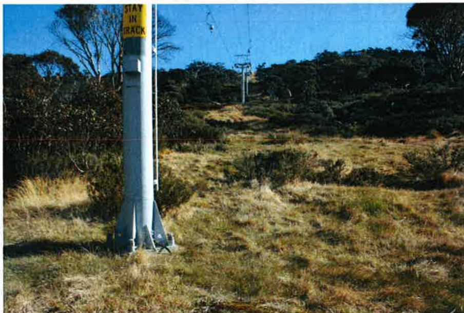
Photograph 3: View upslope with Tower 1 in the foreground.
